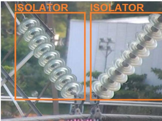
Figure 6 - Visual inspection, isolator identification
