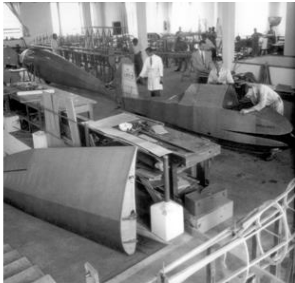
Fig. 11 IPT workshop, gliders construction. [3]
