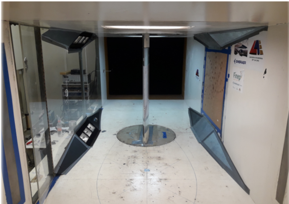
Figure 2 – Installed heating system
