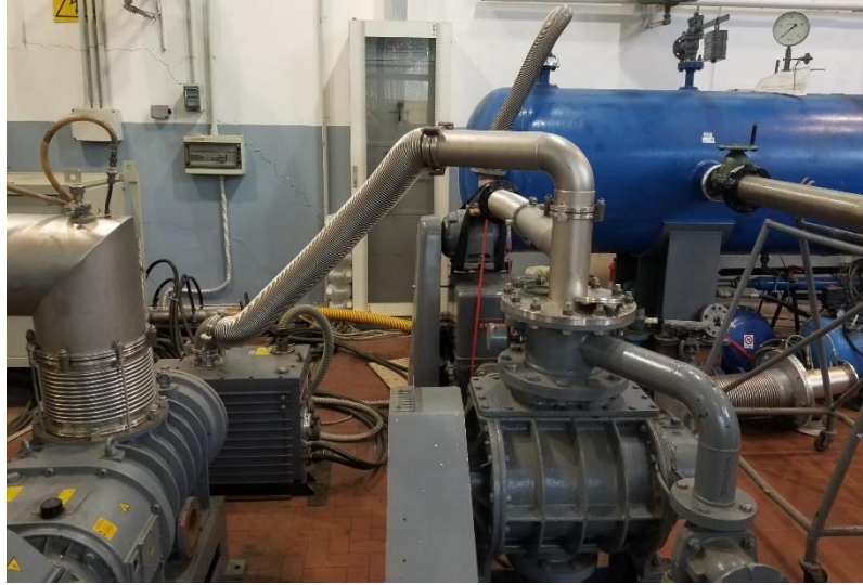
Figure 10 – Vacuum System: (a) Tank, (b) Rotary pumps.
