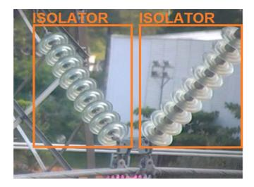
Figure 6 - Visual inspection, isolator identification
