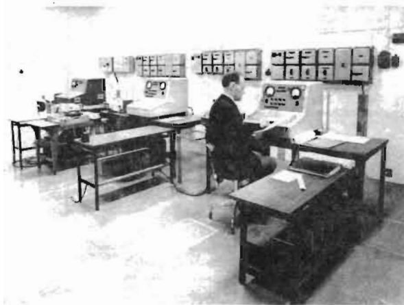
Fig. 2. Digital computer operators' consoles
