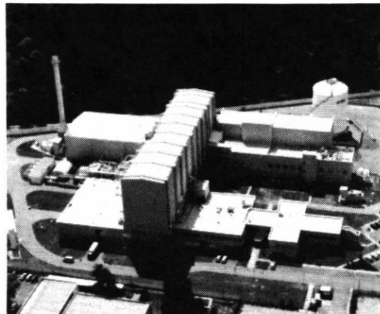
Fig.1 Aerial view of ETW
