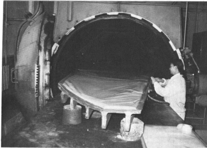
Fig.3 Preparation Work before Curing
