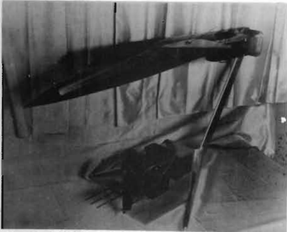
FIGURE 1 WIND TUNNEL MODEL AND FLOW FIELD SURVEY SYSTEM.
